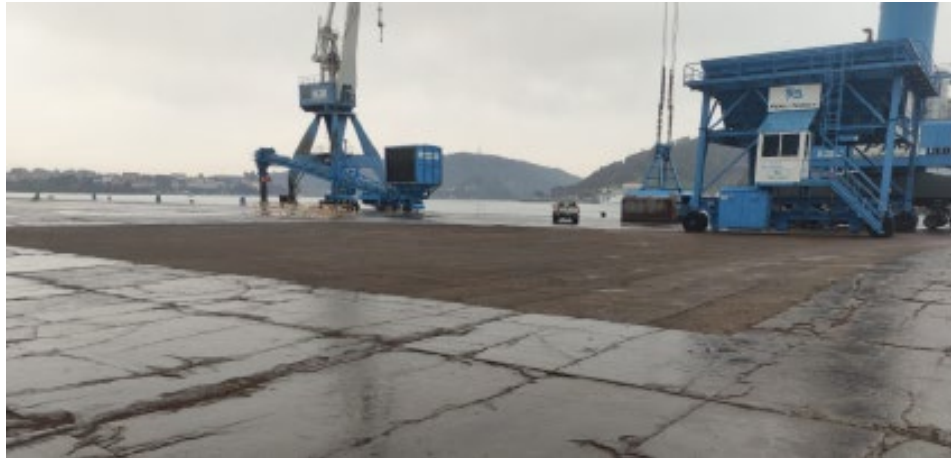
Figure 2. Porous photocatalytic pavement in Ferrol pilot.
